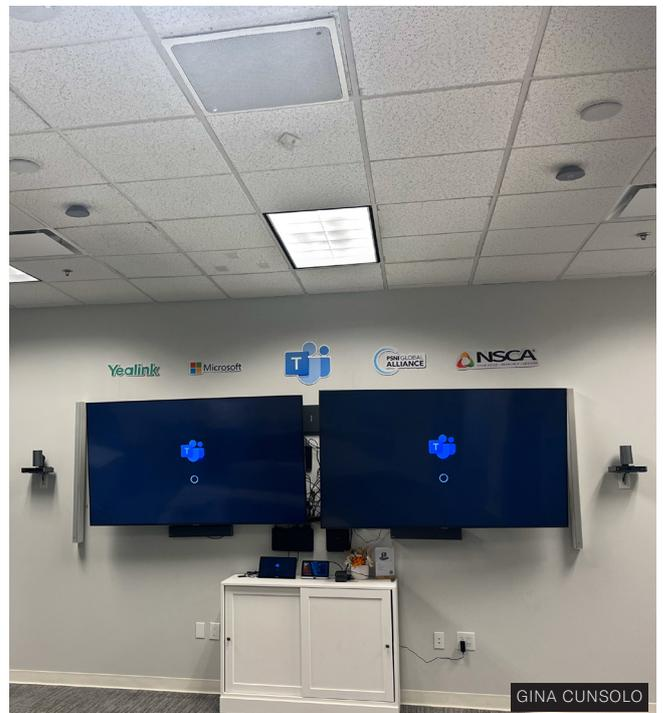
The ADECIA Ceiling Solution delivers crystal clear audio, ensuring every participant's voice is captured with precision. The system's centerpiece is the RM-CG ceiling array microphone, which features four dynamic beams to pick up voices throughout the room. Its advanced adaptive technology adjusts settings in real time, eliminating background noise and echo, enabling natural conversations even in challenging acoustic environments.
